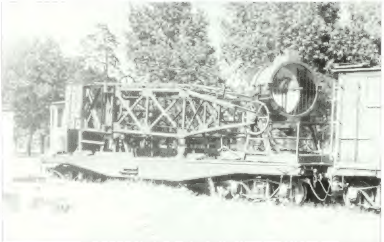
Figure 5.3. Collapsible railway searchlight, no date. Similar to mobile artillery, mobile searchlights as well as small, auxiliary structures were features of Sandy Hook's landscape that played a role in defending the southern approach to New York Harbor. These mobile and sometimes temporary structures will not be addressed in the treatment section (Thomas Hoffman, Fort Hancock , Charleston, SC: Arcadia Publishing, 2007).
